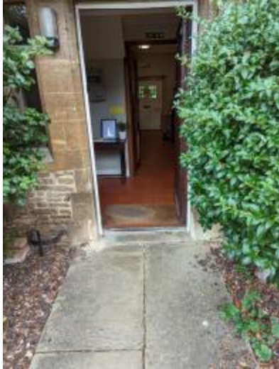
Main front door of Manor House
